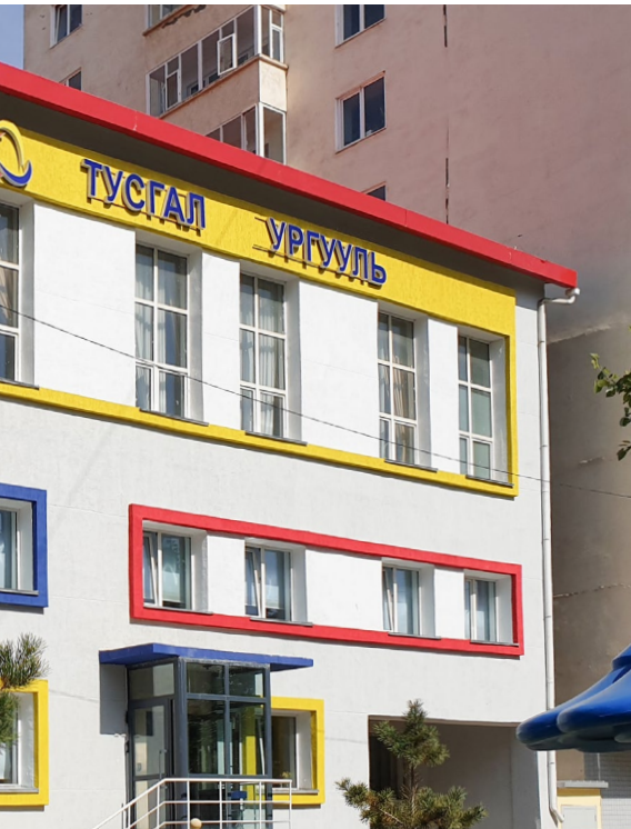
Left: Renovated Tusgal School building
