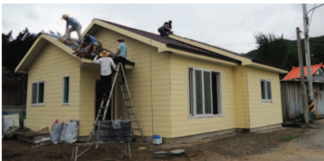
Building experts work on the roof of the new house.
