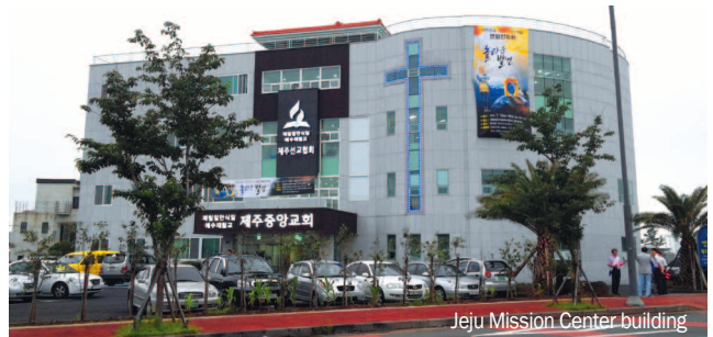
Jeju Mission Center building
